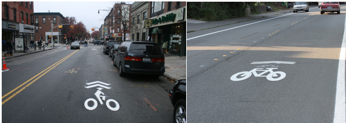
Exhibit 2: Sharrow, a pavement marking installed on streets appropriate for bicyclists but too narrow for conventional bike lanes. The bicycle-plus-arrow markings can be placed in the middle or to the side of the travel lane.
