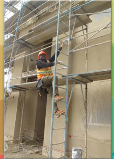
Bryant Collins Jordan Downs Resident Lonestar Construction Journeyman (completed)
