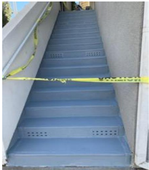
After: Stairs were completely renovated
