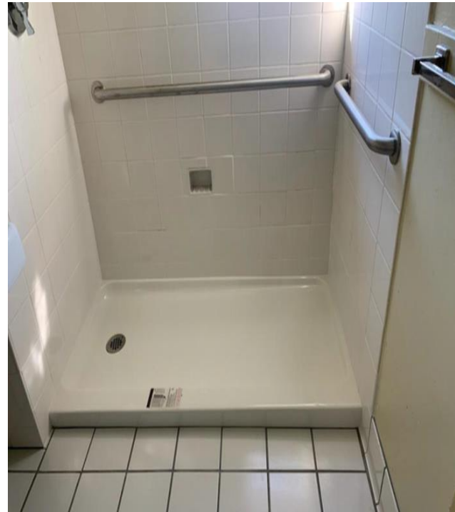
After: The walk-in shower includes grab bars and easier access to get in the shower area
